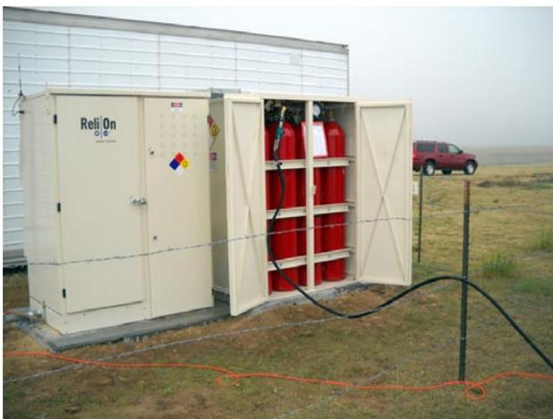
FIGURE 2. Completed AT&T Site (Byers, CO) Undergoing Initial Fill of the HSM
