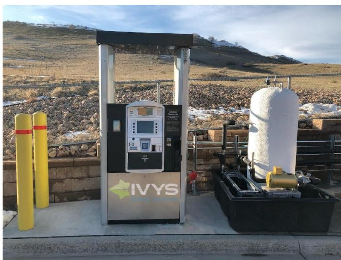
Figure 1. Dispenser and hydrogen cooling system installed at NREL's HITRF
