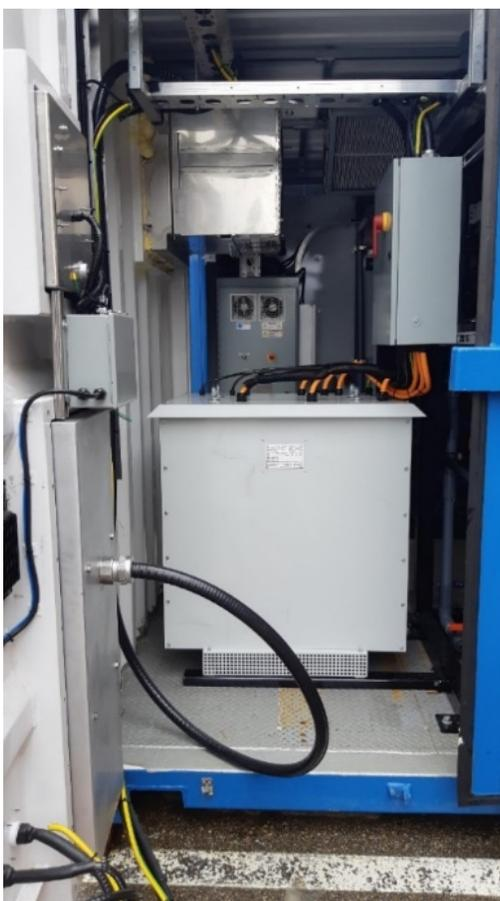
Figure 1. New transformer installed
