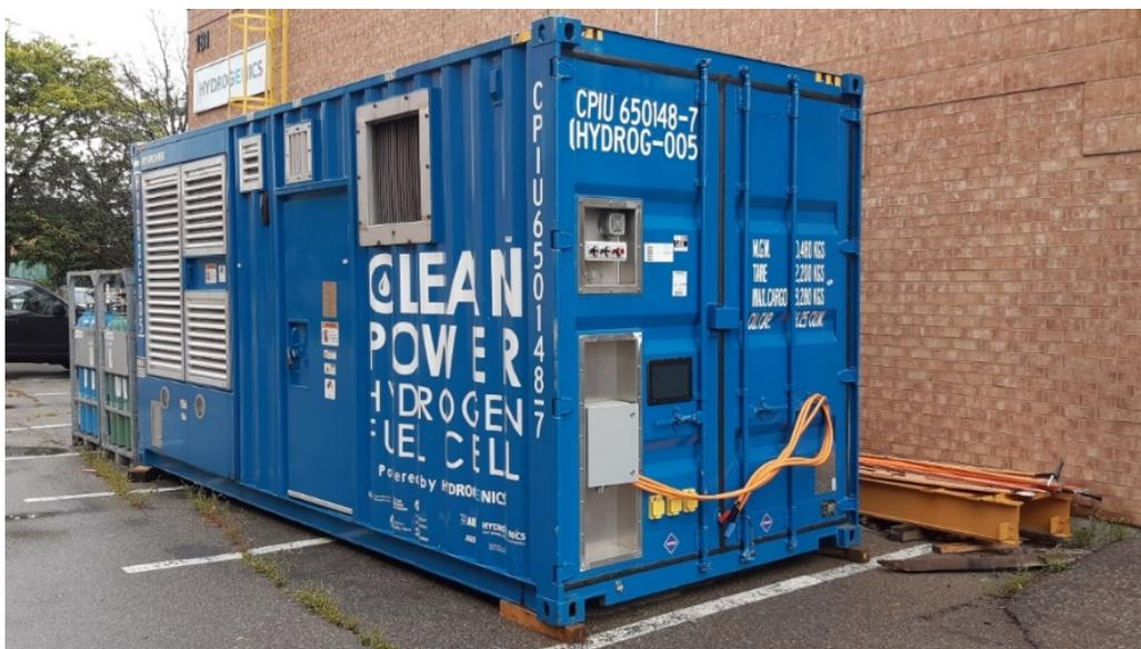
Figure 5. The 100-kW MarFC unit in place for electrical testing at Hydrogenics
