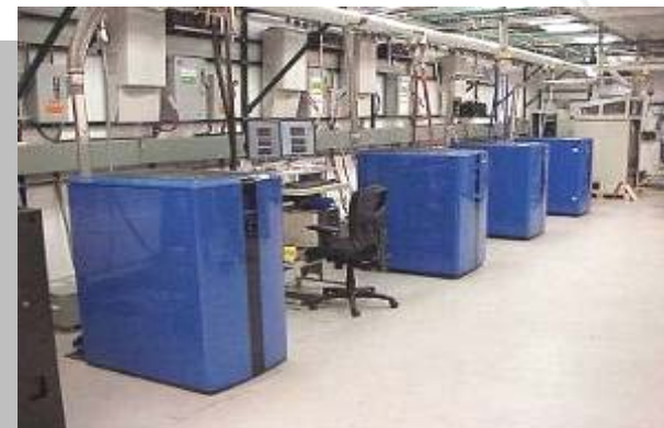
Plug Power Systems Lab
