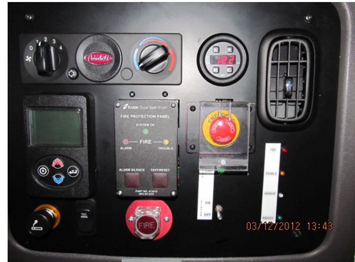
Control Panel Mounted in Sleeper Cab
