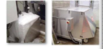
Figure 4. Cold Block and Chiller enable H70 Fast Fill
