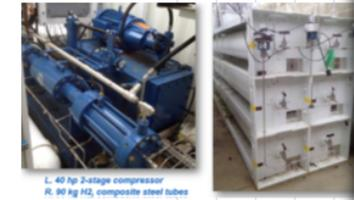
Figure 3. Compression and Storage, SunHydro #1
