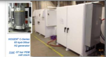
Figure 1. SunHydro #1 Compression, Storage, Dispensing Containerized System
