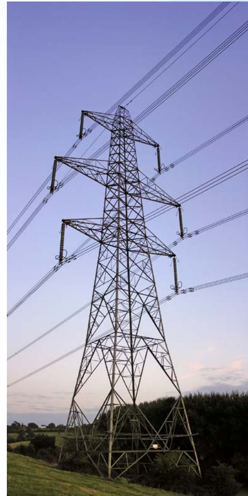
Representative transmission tower. Courtesy of wikicommons.com
