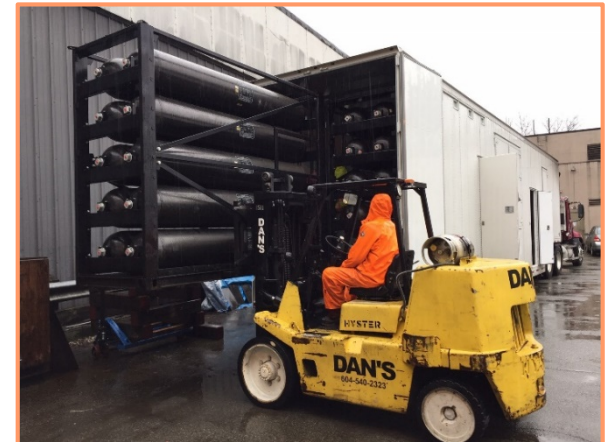
Installation of Powercubes
